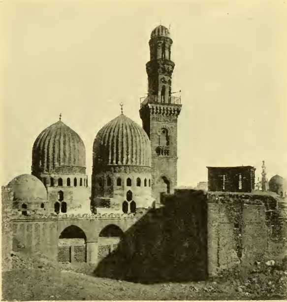
Fig. 69.—Mosque of Sengar and Salār, 1323.
